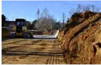
Excavate pipe trench and lay inlet pipe to required fall and invert level. Install silt traps in appropriate locations in pipe run if not using ACO StormBrixx® access chamber, sediment tunnel or forebay.
