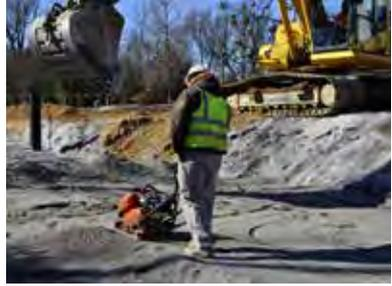
**Top** - Use a minimum 4" (100mm) coarse sand protection layer over top of ACO StormBrixx® units and geotextile then backfill. A minimum 16" (400mm) backfill cover is required before compaction equipment is used. Area should be compacted using suitable compaction equipment.
