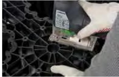
Place an inspection point connector over center of hole, ensuring flange covers all four columns. Using plastic rivets, fix flange to StormBrixx® unit. If an extension piece is required, use 9" (225mm) dual wall pipe cut to length and attach with proprietary coupling.
