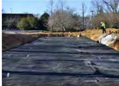
Complete encapsulation by wrapping protective fleece horizontally around tank and tape into position.
